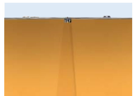
The relatively narrow gap is closed by the jockey cover. (pattern matching possible)
